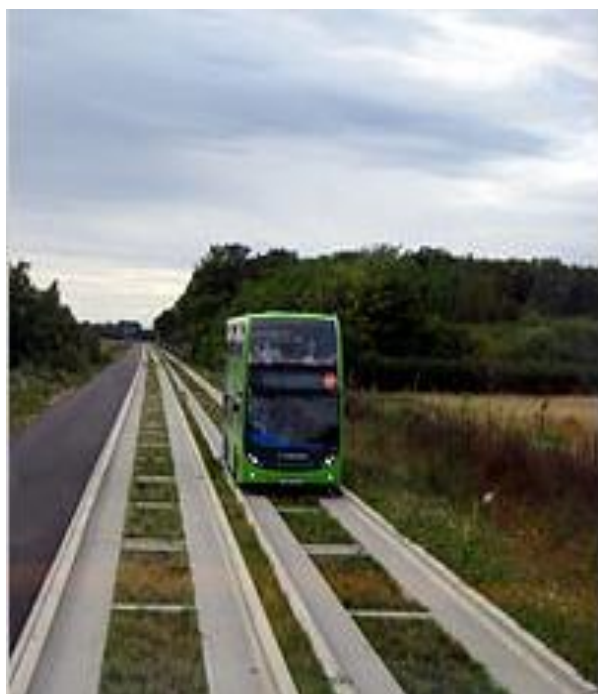
The busway between Oakington and Longstanton. The cycle path runs alongside on the left.
